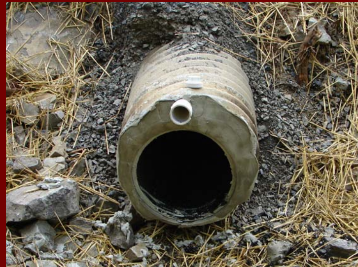
Step 7: Seal ends and install PVC pipes
