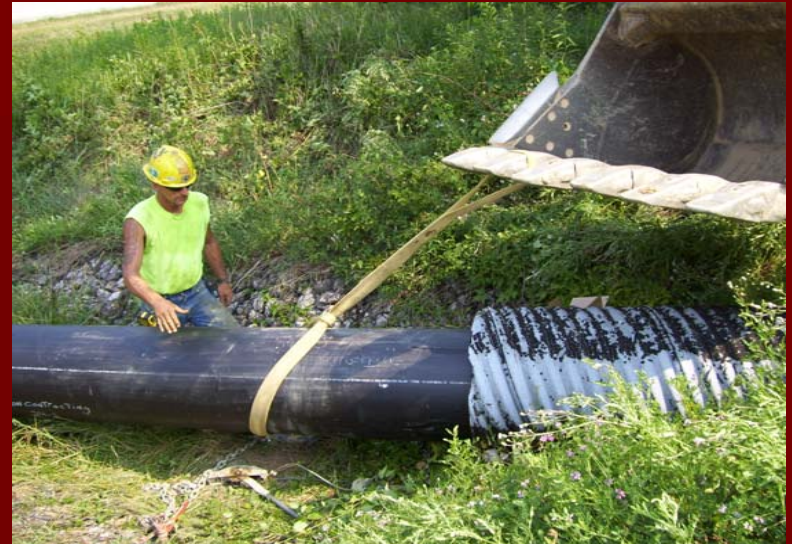
Step 7: Seal ends and install PVC pipes
