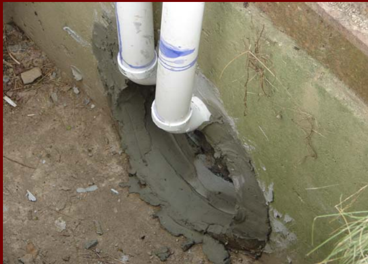
Step 7: Seal ends and install PVC pipes
