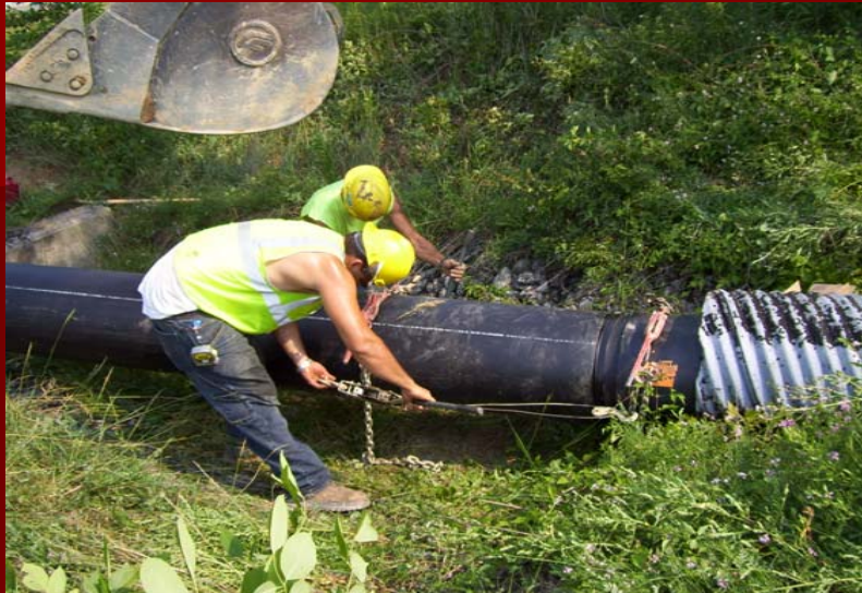
Step 7: Seal ends and install PVC pipes
